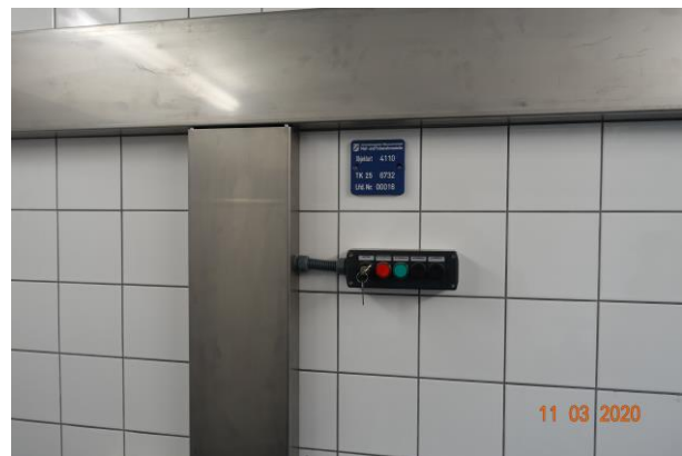
Detail: E-Installation Brunnenstube – VOS
